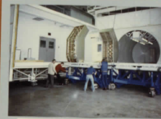
Experiment racks placed into position for installation into Spacelab Mockup
