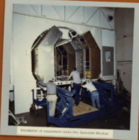
Installation of experiment racks into Spacelab Mockup
